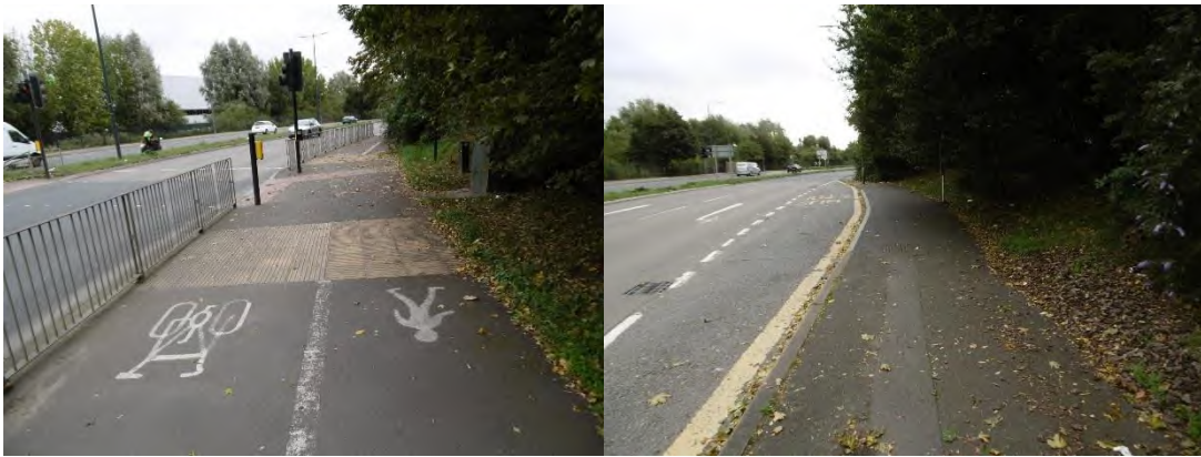
Figure 2.3 Pictures of Picardy Manorway Westbound
