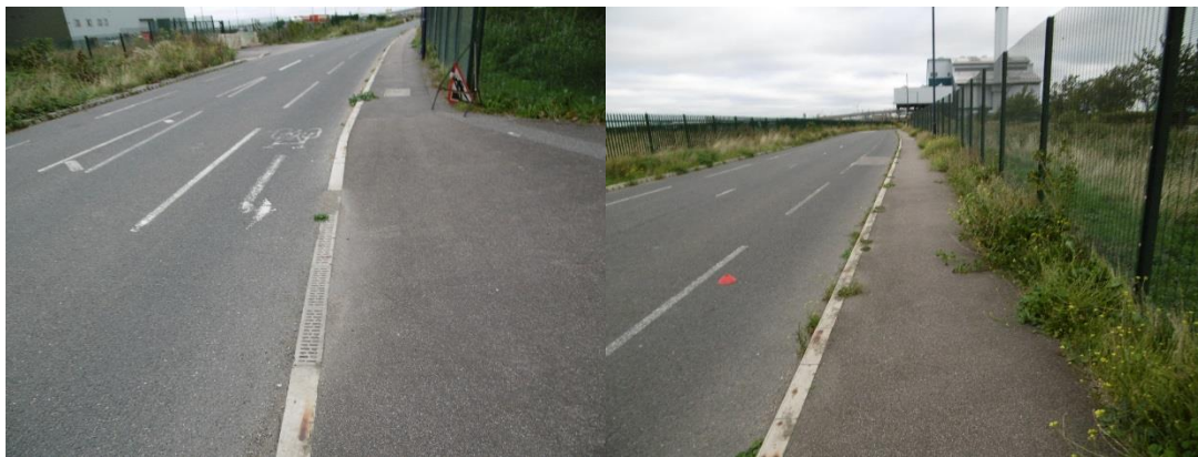
Figure 2.1 Pictures of Norman Road (north of Picardy Manorway)
